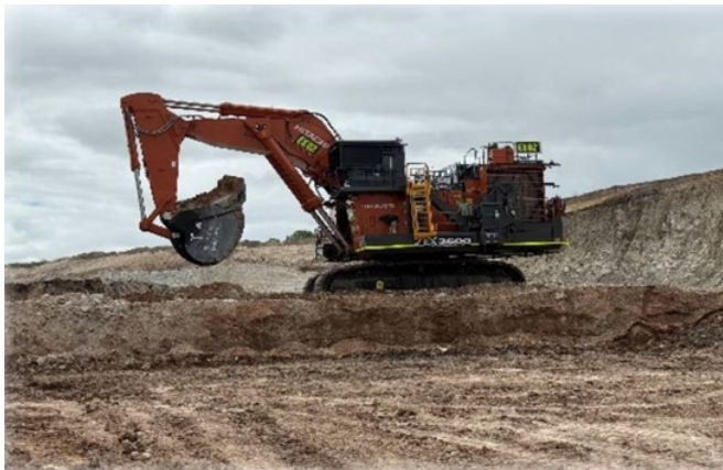
New EX3600-7 – First Bucket of Dirt
